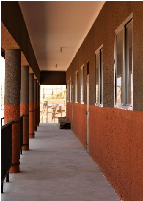
A view of the corridor outside one of the classrooms. A disabled access ramp has been provided
